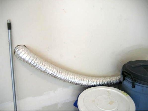
Another best practice is to restrict the dryer exhaust duct from passing through an attached garage. Ducts in the garage or penetrating the walls or ceilings separating the dwelling from the garage must be constructed of minimum No. 26-gauge sheet steel or other approved material, having no openings into the garage.
