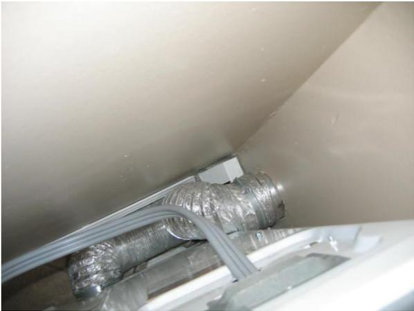
The transition duct (the visible piece of duct connecting the dryer to the wall area) can be up to 8 feet long and should be listed in accordance with UL-2158A. There are some semi-rigid metal transition duct products that are UL-listed. Transition ducts must be visible and not concealed within construction.
