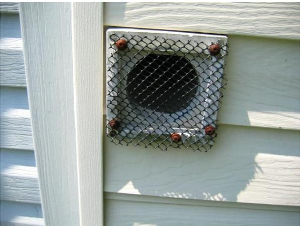
The exhaust duct should terminate outside the building at least 3 feet from any building opening, and at least 10 feet from an air conditioner or heat pump condenser. The duct termination should be fitted with a closeable gravity or automatic damper (a backdraft damper). A screen may not be installed at the duct terminus (2009 IRC M1502.3), as it can trap debris, which poses a fire hazard.
