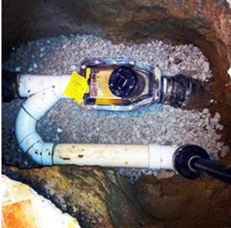
**Installing a backwater valve will prevent sewer drains from backing up and overflowing with sewer water – eliminating sewer backflow as a source of basement flooding.**
